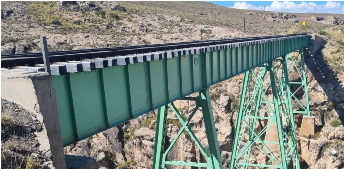
Figura 27: Vista general Celosía
