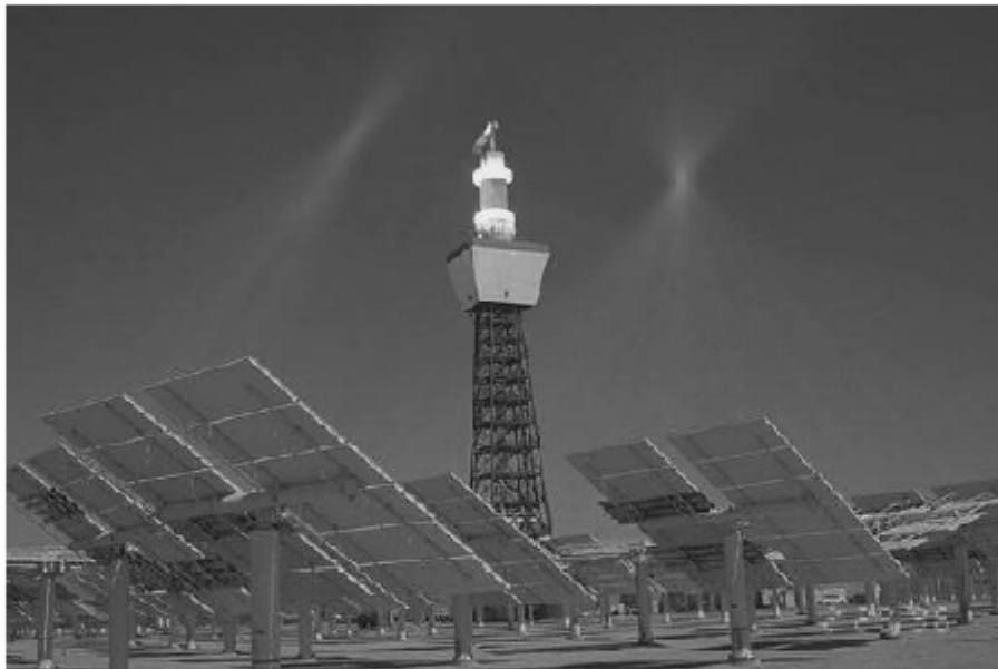
Figure 1. The Solar Power Tower at Barstow, CA
