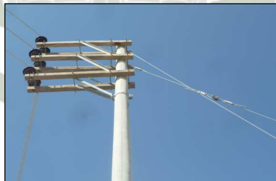
Figura 42: Retenida defectuosa
