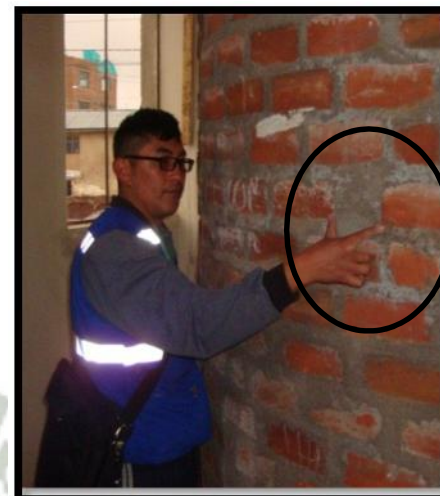
Figura 35. Junta mayor a 2.5mm
