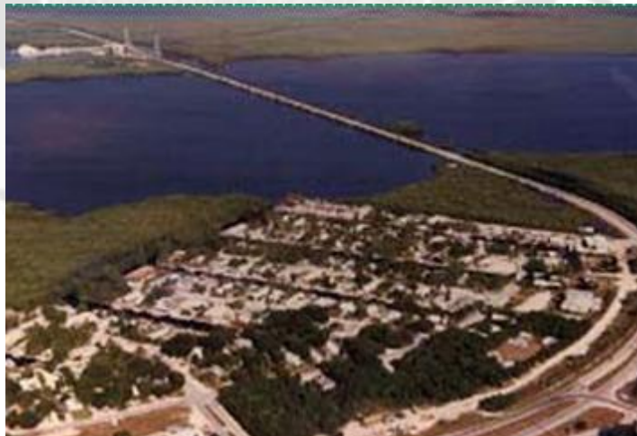
Figura 3.12 Puente Jewfish Creek. Florida, USA
