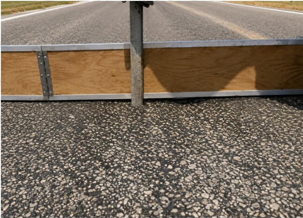
FIG. X1.42 Medium-Severity Rutting
