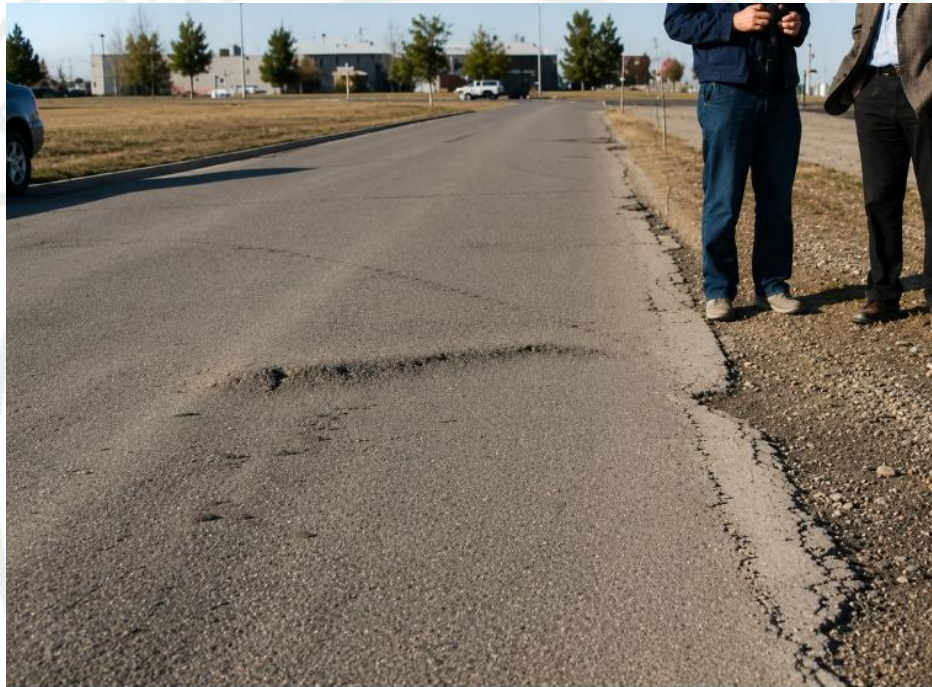
FIG. X1.11 Medium-Severity Bumps and Sags
