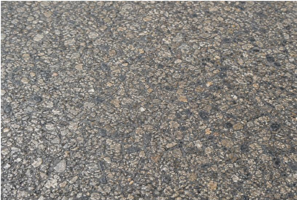
FIG. X1.34 Polished Aggregate
