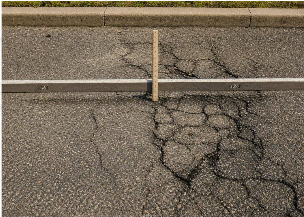
FIG. X1.18 High-Severity Depression
