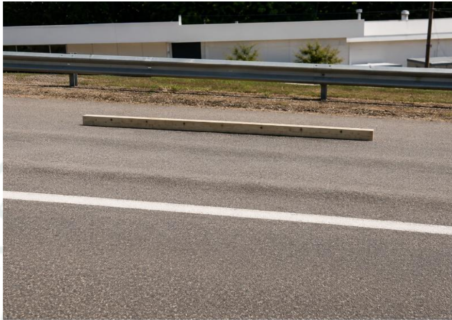
FIG. X1.14 Medium-Severity Corrugation
