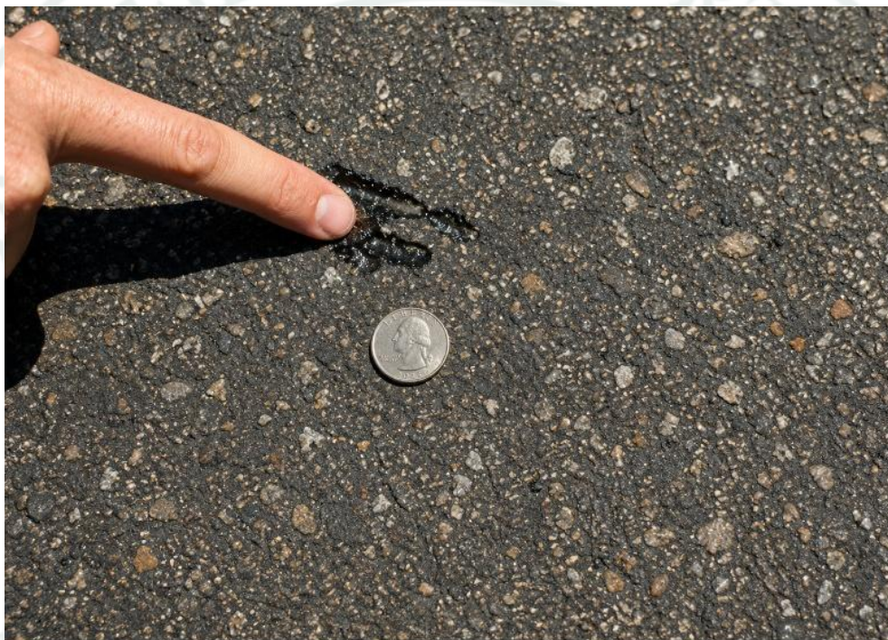
FIG. X1.5 Medium-Severity Bleeding
