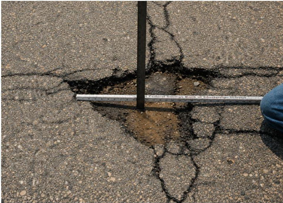
FIG. X1.36 Medium-Severity Pothole
