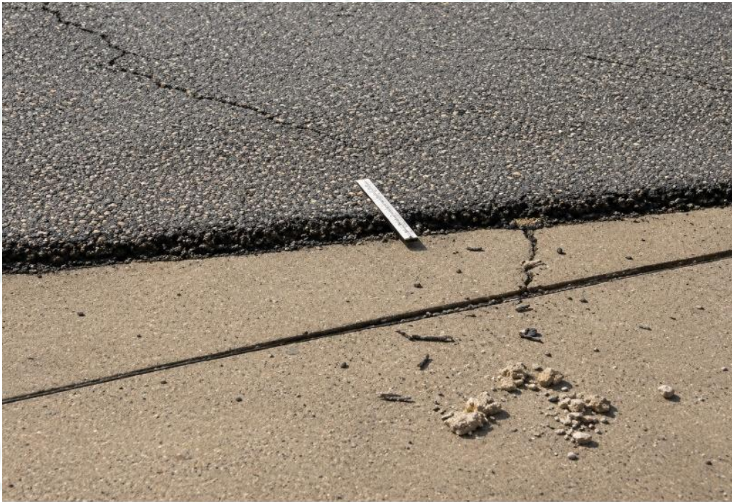
FIG. X1.45 Medium-Severity Shoving
