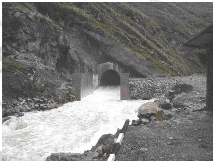
Figura 2.6 Decant Tunnel Antamina – Perú (2016)
